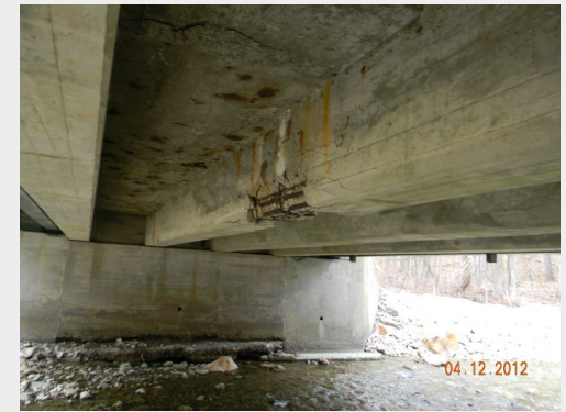
Exposed Rebar
